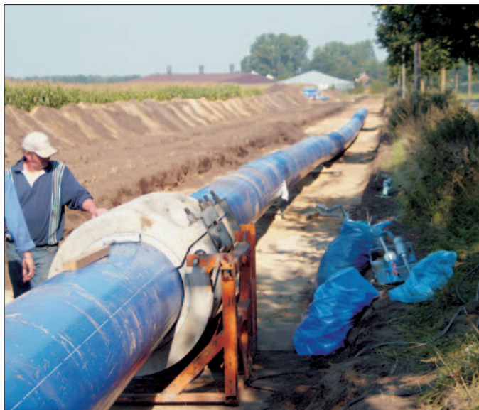
Fig. 5: Welding of two prepared pipe strings
